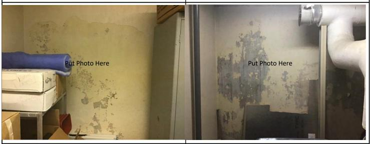
Damage Description:Item #:81Damage Description:Item #:82Wall, drywall, repair, cracked, caused by rainwater intrusion (Main Bldg., Basement, Laboratory R029 & 028)Ceiling, drywall, painted, cracked, caused by rainwater intrusion (Main Bldg., Basement, Laboratory R028 & 029)Additional Comments:Additional Comments:
