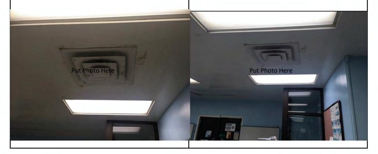
Damage Description: Damage Description: Item #: 164 Item #: Ceiling, drywall, paint, discolored and moldy above, caused by Window, Alum. window frames, perimeter caulking/sealing only, rainwater intrusion (Main Bldg., Floor 1, Laboratory R094) cracked, caused by wind-driven rain (Main Bldg., Floor 1, Office R067) **Additional Comments:**
