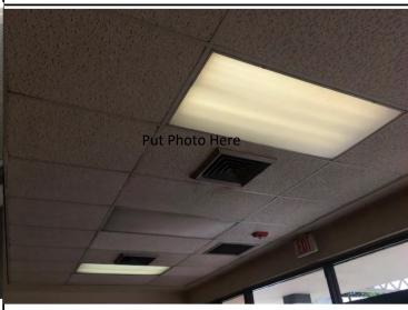
Damage Description: Item #: Ceiling, 2 FT x 4 FT acoustic tile, suspended, grid only, dislodged, caused by rainwater intrusion (Main Bldg., Floor 1, Entrance Lobby) Damage Description:
