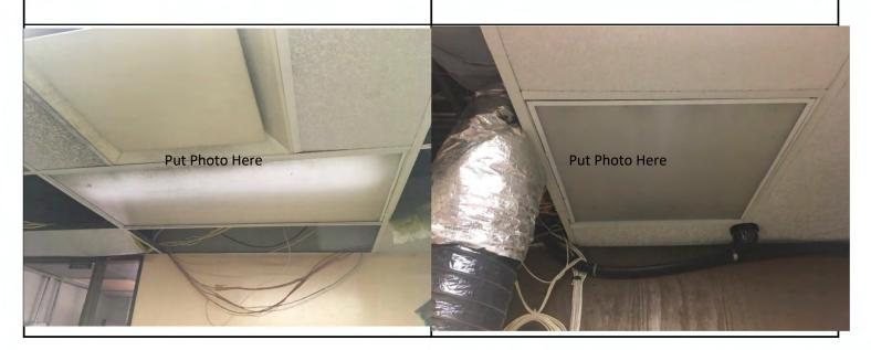
Damage Description:Item #:120DarLight, fluorescent, recessed Troffer, acrylic prismatic lens only,<br/>deformed, caused by rainwater intrusion (Main Bldg., Floor 1, Server<br/>Room)Urel<br/>Bldg
