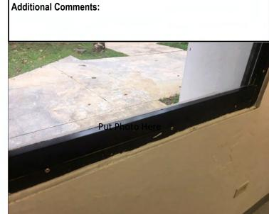
Window, Alum. window frames, perimeter caulking/sealing only, cracked, caused by rainwater intrusion (Main Bldg., Floor 1,
