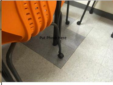
Floor, VCT, 12x12 IN, dislodged, caused by surface water
